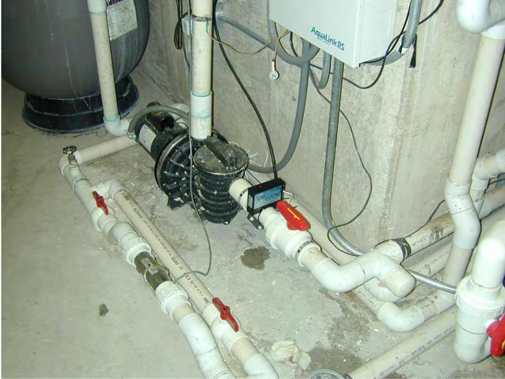
Photograph of installed *HydroFLOW* water conditioner
