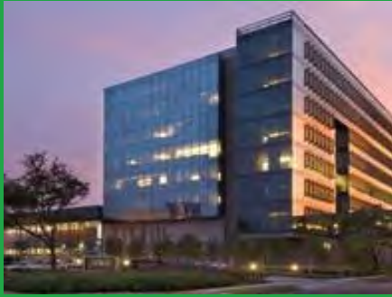
LEED Gold Headquarters Building Houston, Texas 1,000 Ton Cooling Tower
