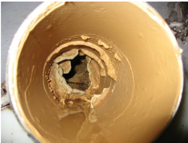
Untreated D1 nozzle – close up
