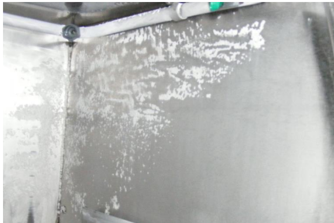
6 months after installation
