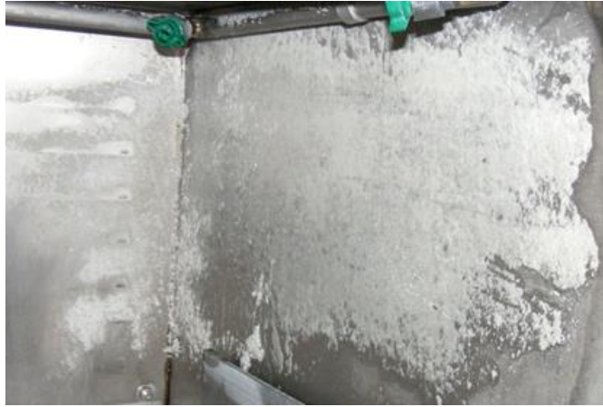
Prior to installation
